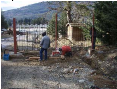
Gates being installed off Bell McKinnon Rd
